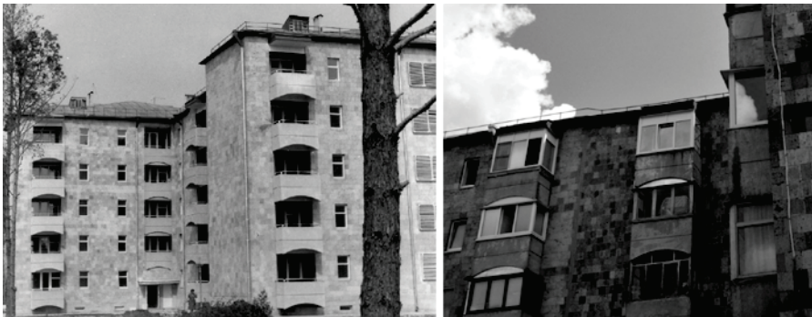
Fig. 9: Initial look of the blocks in Yerevan quarter and contemporary variations of window frames in the Yerevan quarter (wooden and “Eurowindows,” perfect-fit and rectangular forms). Photos: left—Yevhen Alimov Collection; right—Studio Collection, Archive of the Center for Urban History
